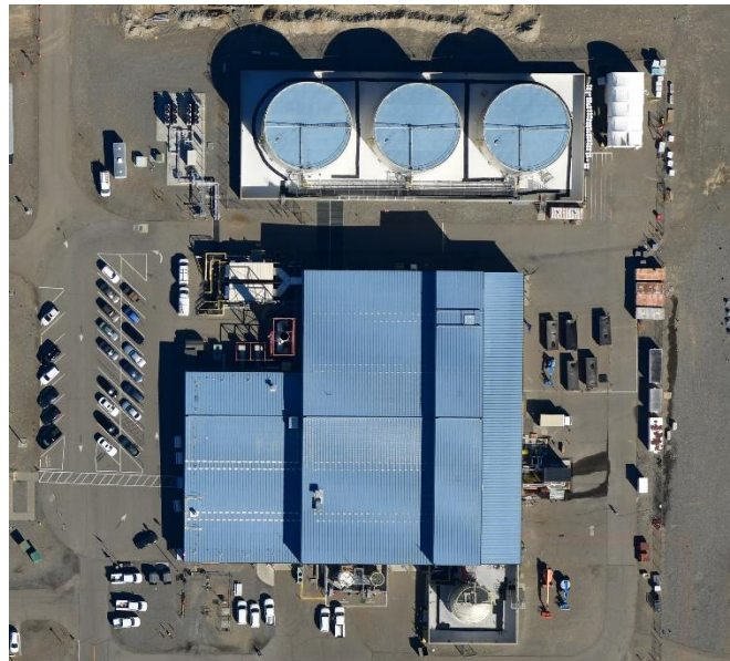
An aerial view of the Effluent Treatment Facility in the 200 East Area
