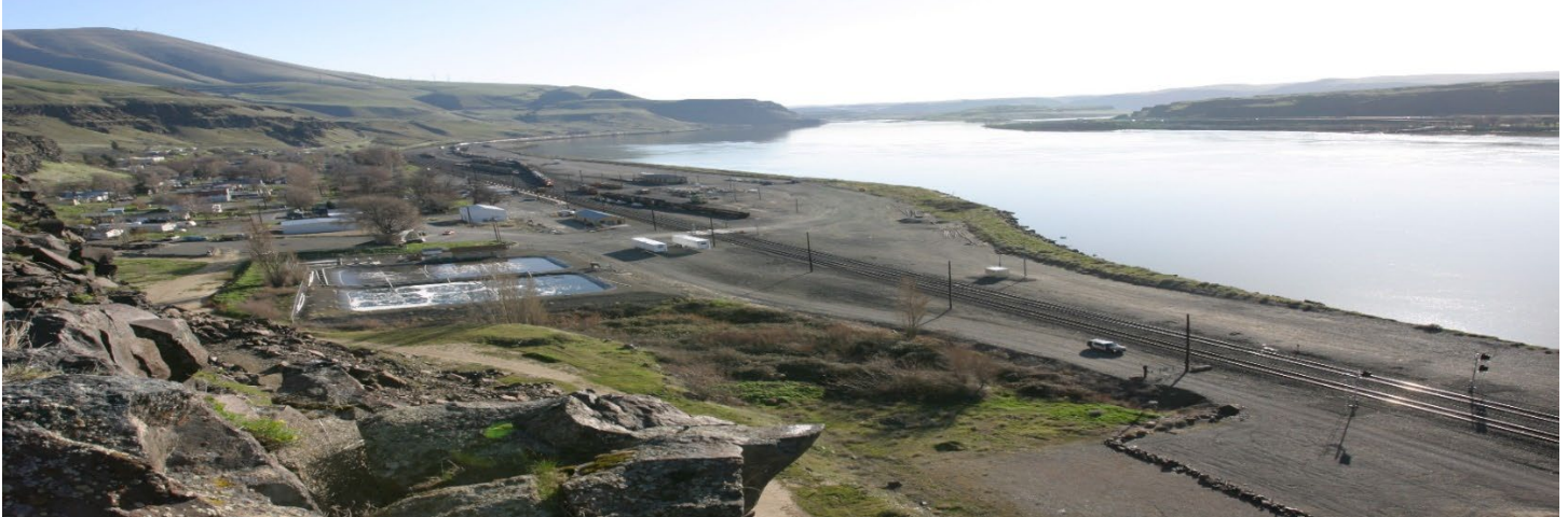
BNSF Track Switching Facility aka Wishram Site
