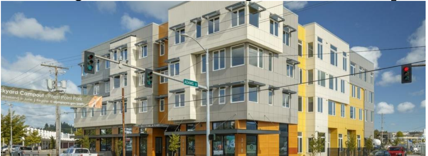
Figure 1. The Billy Frank Jr. Place, a former cleanup site, offers affordable housing. Photo: Housing Authority of Thurston County.
