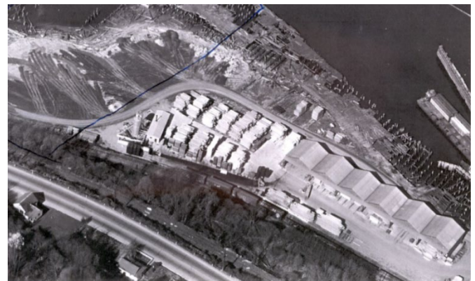
Aerial view of RG Haley site operations, 1953
