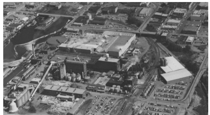
Lignin warehouse (light-colored roof on right) and storage tanks, 1974
