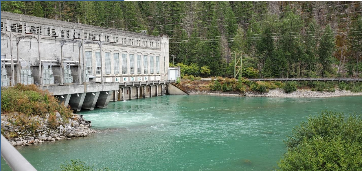
Gorge Power Plant on Skagit River
