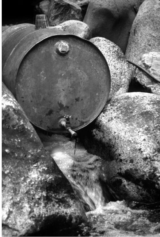
FIGURE SOP 7.2. Dispensing liquid 2% \text{KMnO}_4 solution into the main flow of a stream. Note the manually controlled spigot for controlling the flow of the solution and the large stoppered hole used for filling the dispensing barrel.
