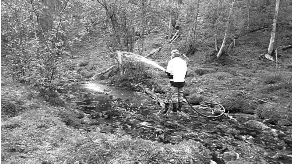
FIGURE SOP 13.2. Applying Vectocarb/CFT Legumine slurry with portable water pump and garden hose in upwelling groundwater area.
