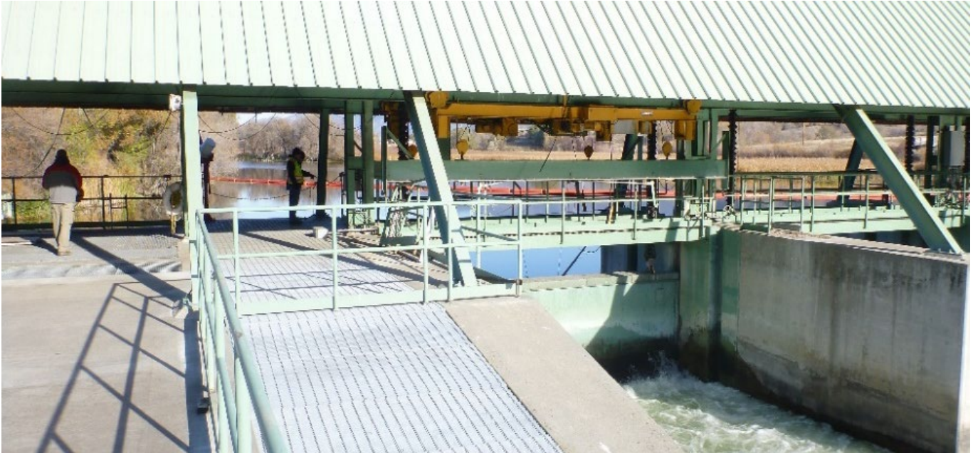
Figure 1. Zosel Dam, Okanagan County, engineers at work
