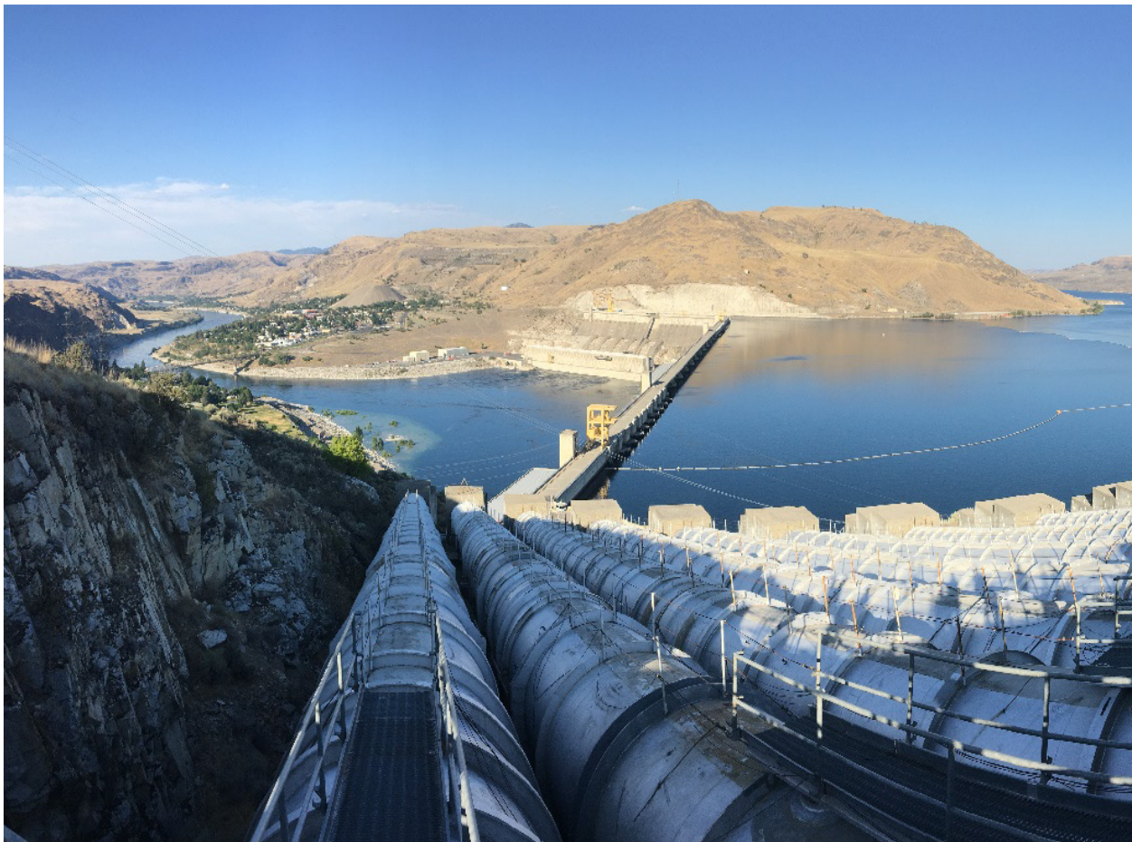
Pipes moving irrigation water from Lake Roosevelt at Grand Coulee Dam to Banks Lake Photo Credit: Tom Tebb, 2018
