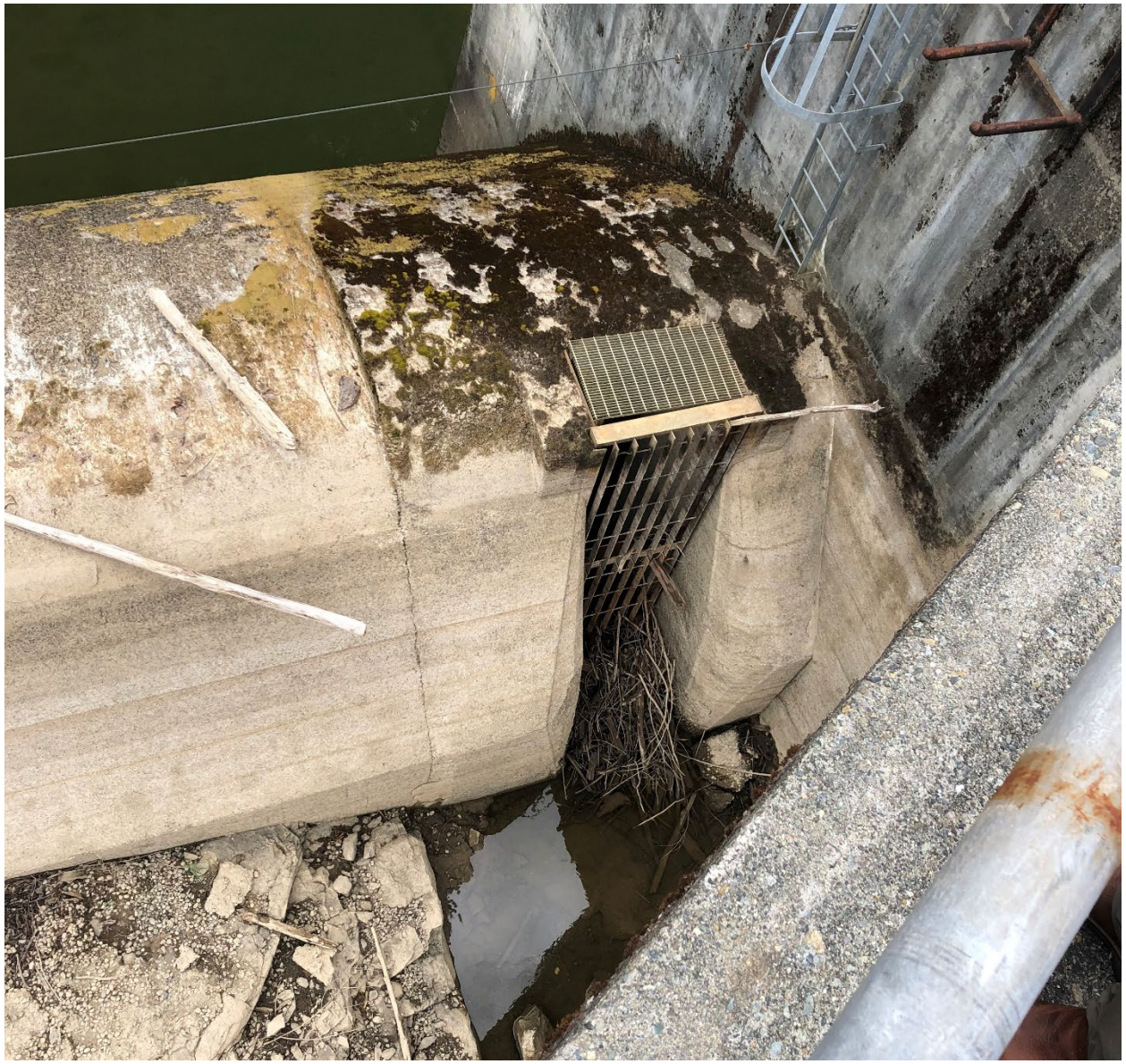
Figure 3 Photograph of Fish Sluice in Spillway
