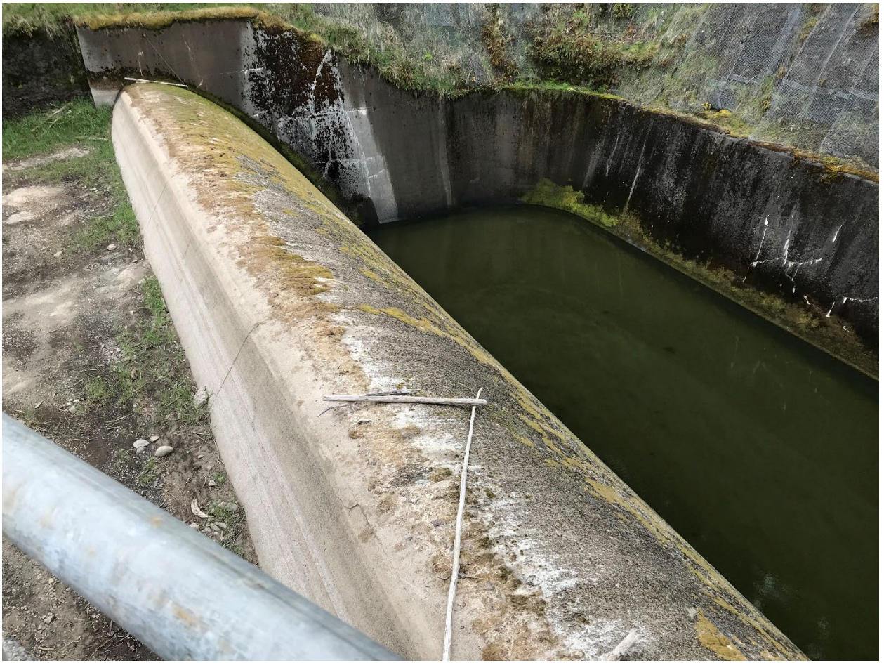
Figure 2 Photograph of Spillway
