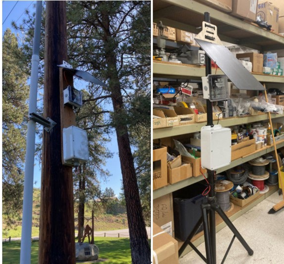
Figure 6: Pictures of SensWA with Voltaic solar power systems
