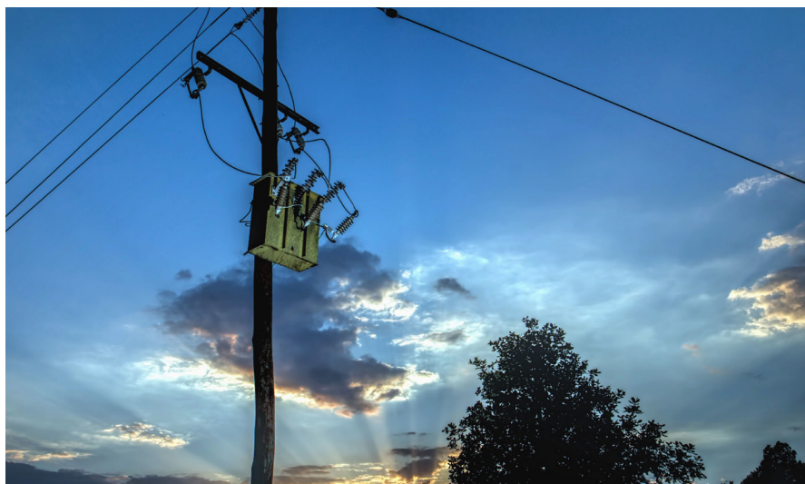
Figure 5. One example of WPCBs is transformers that contain PCB fluids with concentrations greater than or equal to 2 ppm.
