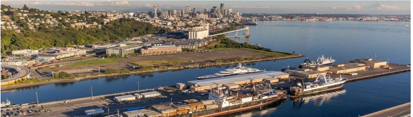
Aerial view of Terminal 91 on Elliot Bay in Seattle
