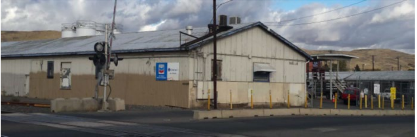
Coleman Oil Yakima Bulk Plant
