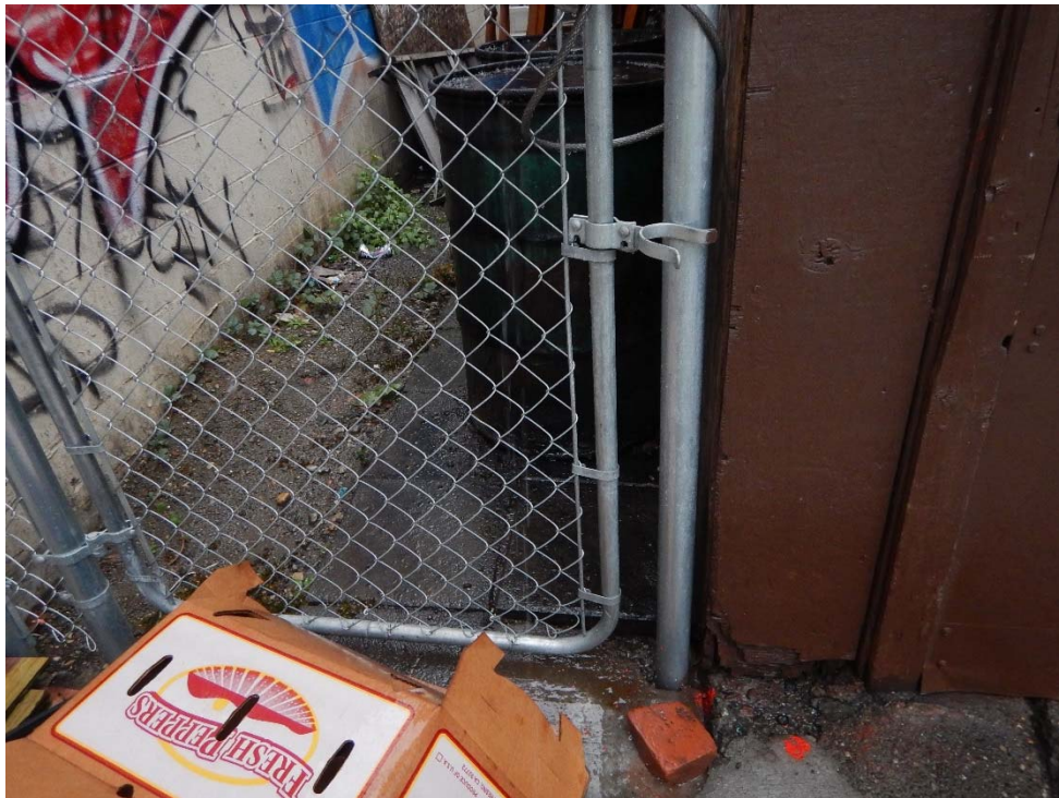
Photograph 2: View of fenced alley and Building Addition, facing east. Orange paint marks the continuation of Pipes 2 and 3 identified by the utility locator. The locate marking for Pipe 1 was located directly north of the red brick in view, but was obscured by heavy rainfall.
