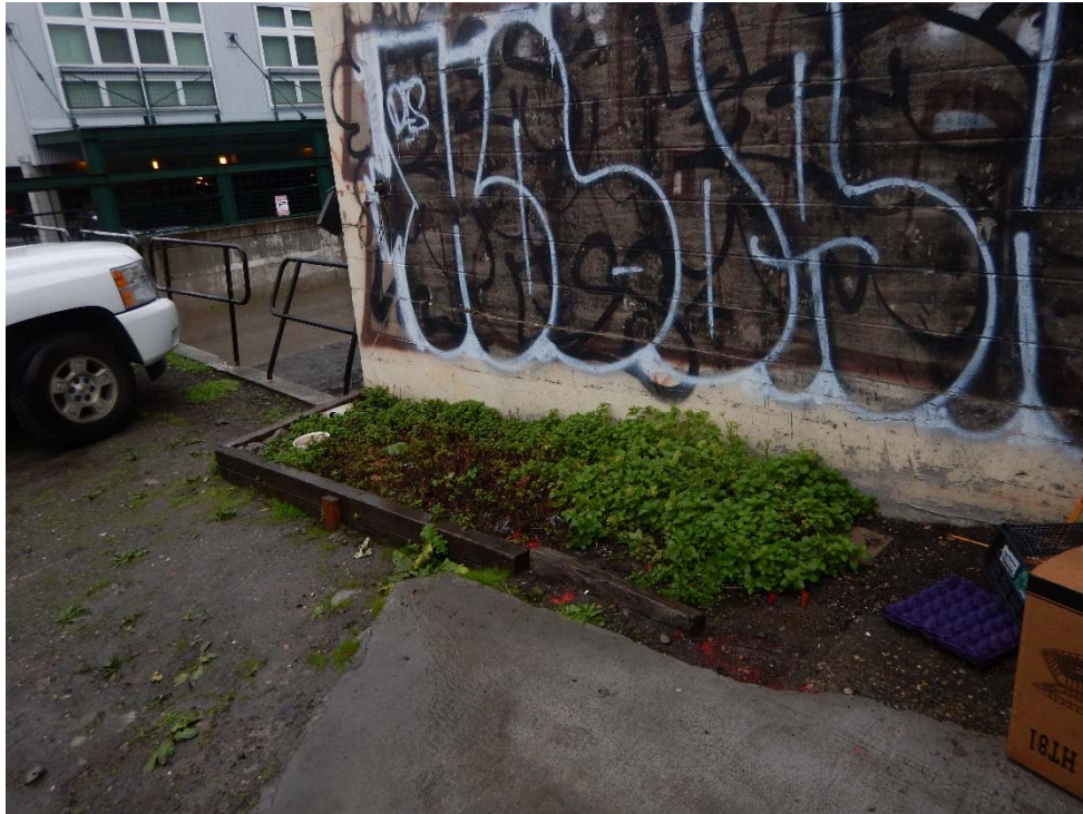
Photograph 1: View of excavation area, retaining wall, and Jurgensen building prior to excavation activities, facing northwest.
