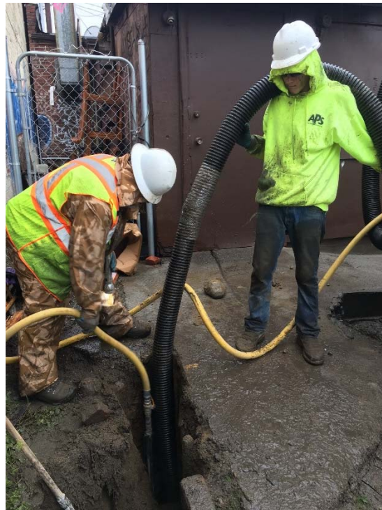
Photograph 4: Excavation in progress adjacent to Pipe 3, facing east.
