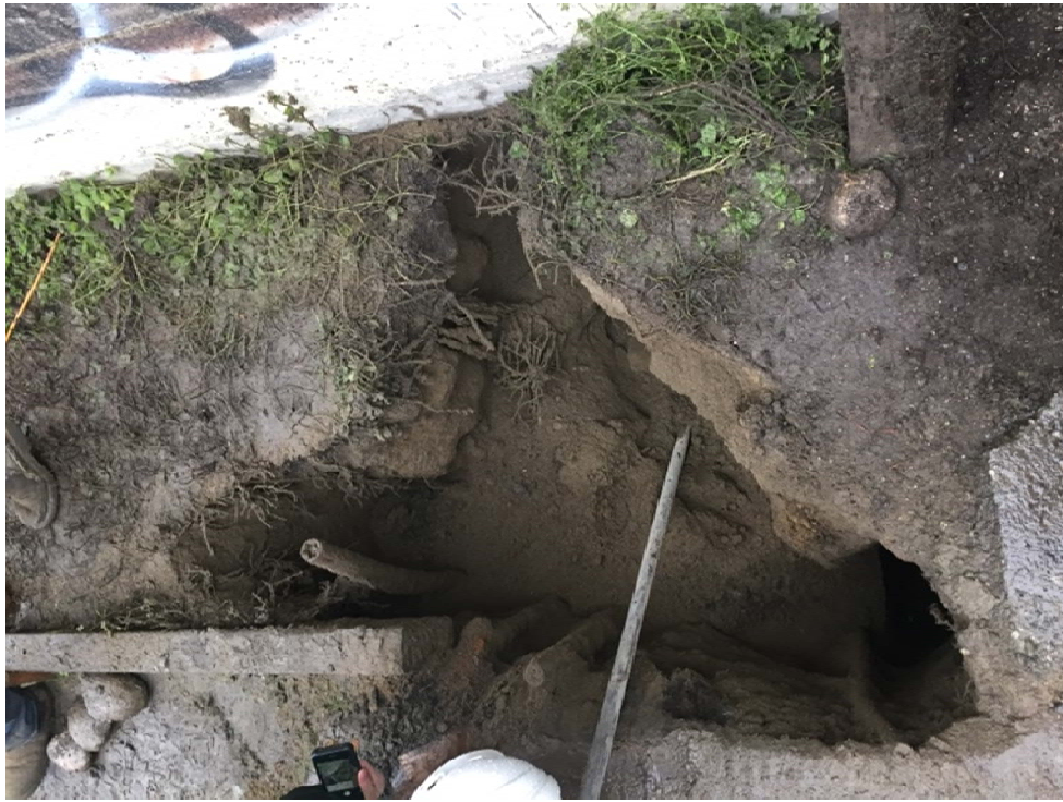
Photograph 7: View of total extent of the excavation, with the Jurgensen building retaining wall in view.
