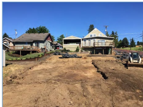
Figure 18: Soil replacement on a property
