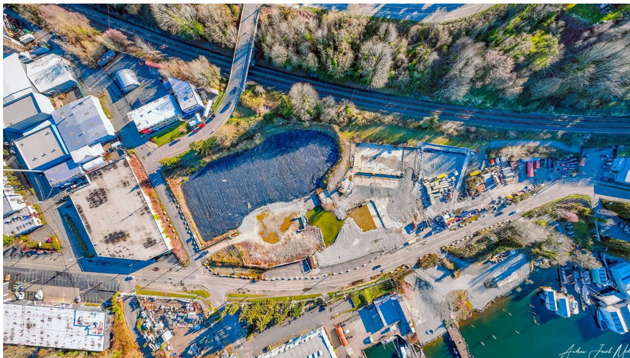
Figure 17: Aerial view of post-remedial construction conditions
