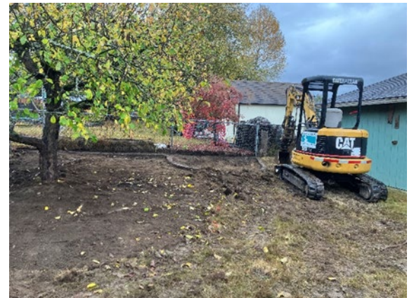
Figure 6: Soil excavation in spring 2023
