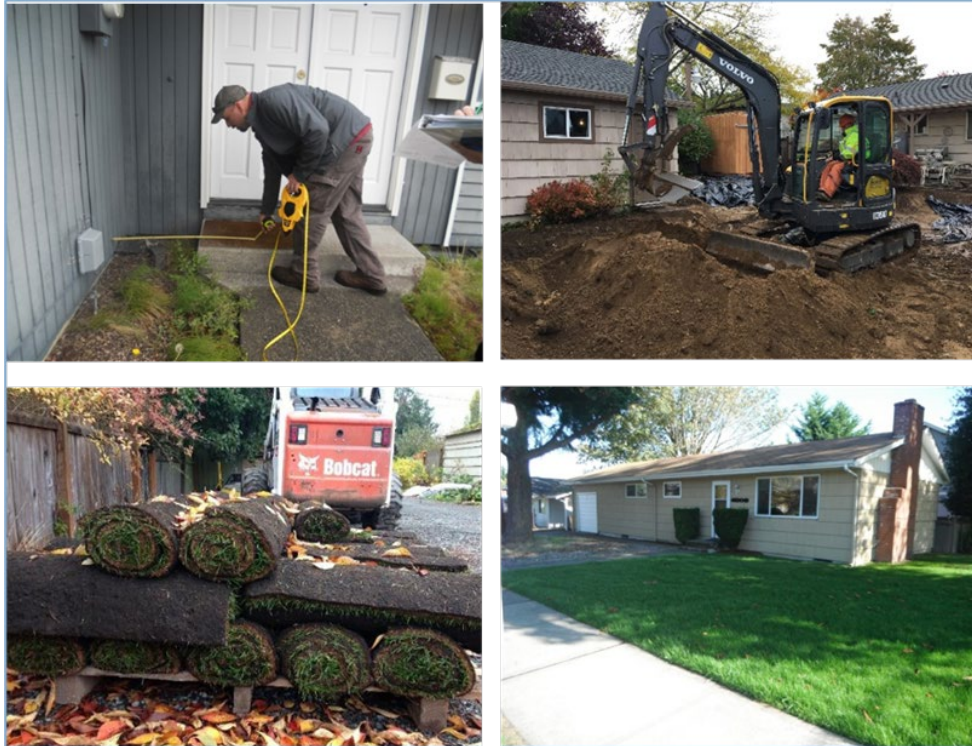
Figure 8: Steps towards soil replacement
