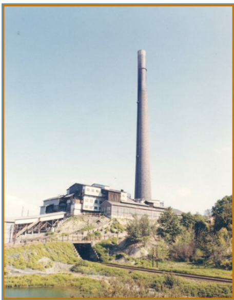
Figure 2: Tacoma Smelter Plume smokestack
