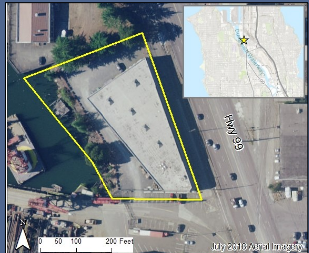
Aerial View of Snopac Property
