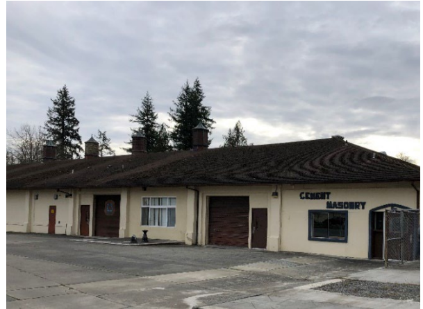
AOC 1, Former Laundry Building, January 2019
