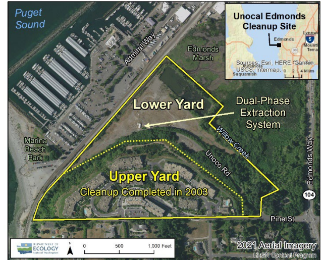
Aerial view of Unocal Edmonds site
