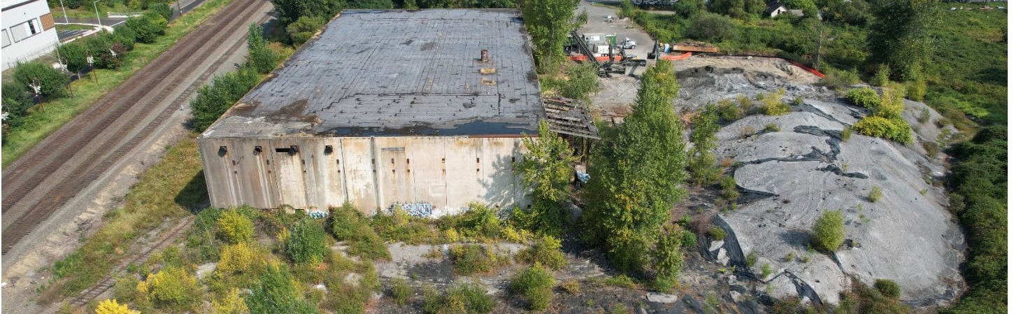
Maralco site aerial photo (2023)
