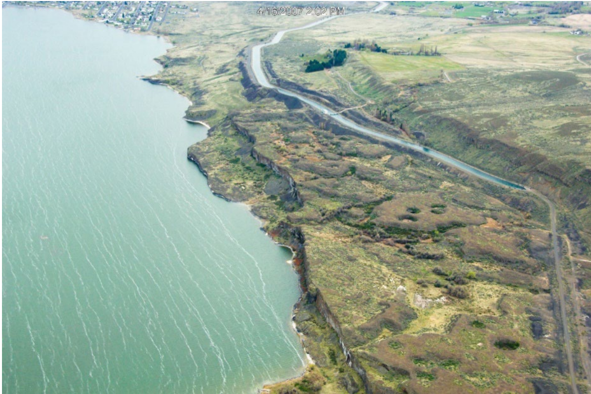
Figure 5 Irrigation water flows from Soap Lake Siphon (lower right) into West Canal along western side of Soap Lake (Image: Ecology, 2007)
