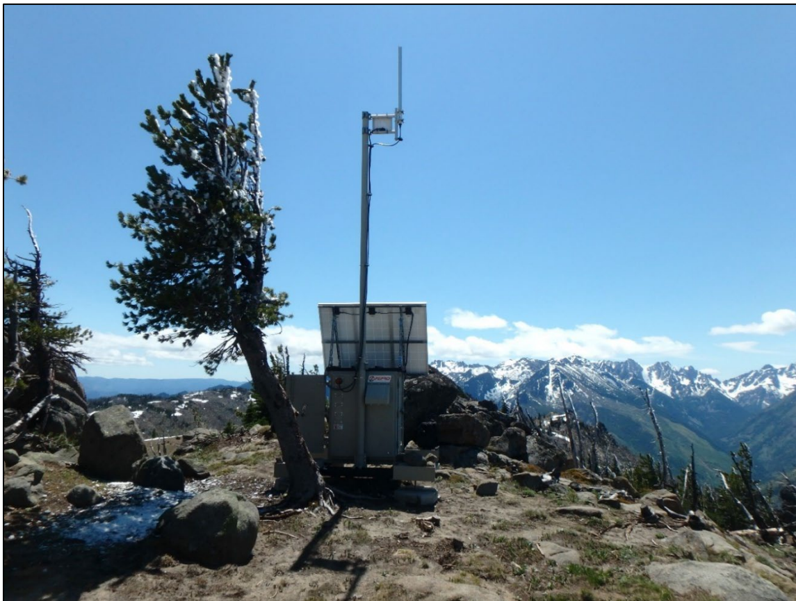
Figure 2-10. Forest Service Icicle Repeater Station
