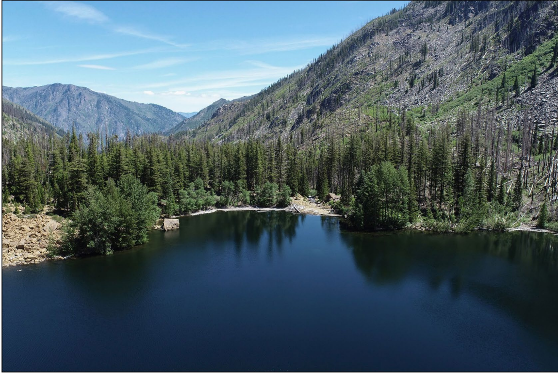
Figure 11-19a. View of Existing Dam from KVP C (water level approximately 4,667 feet)
