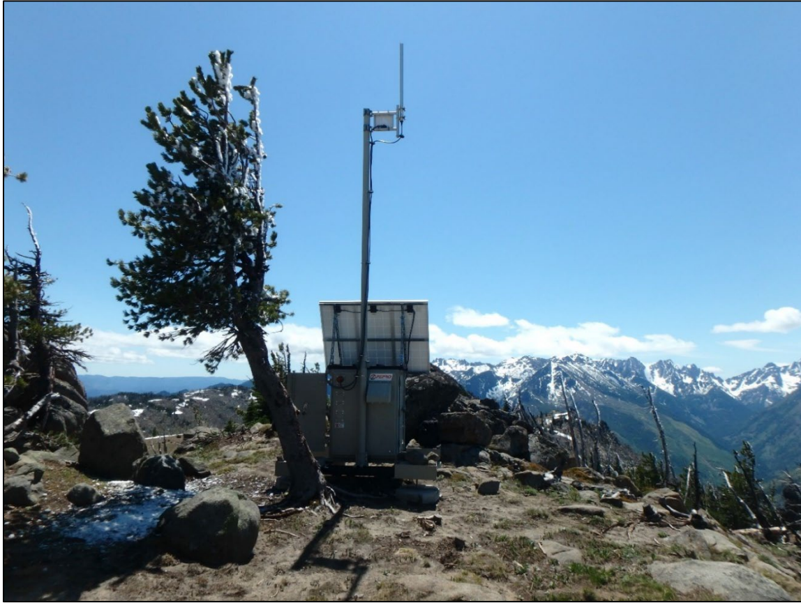
Figure 9. Forest Service Icicle Repeater Station
