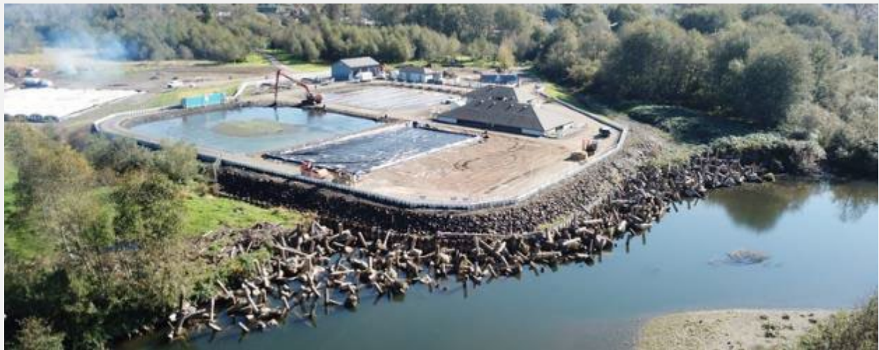
Log jacks on the Wynoochee riverbank protect the Montesano Wastewater Treatment Plant. Photo credit: Parametrix
