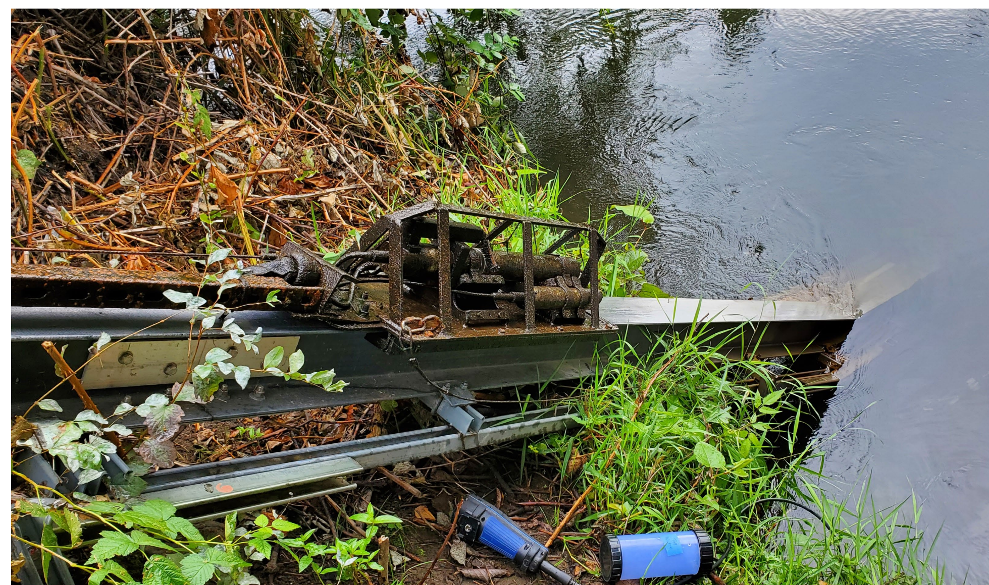
Figure 1. The Duwamish River (09A075) I-beam shuttle and sensors removed from the water for cleaning.
