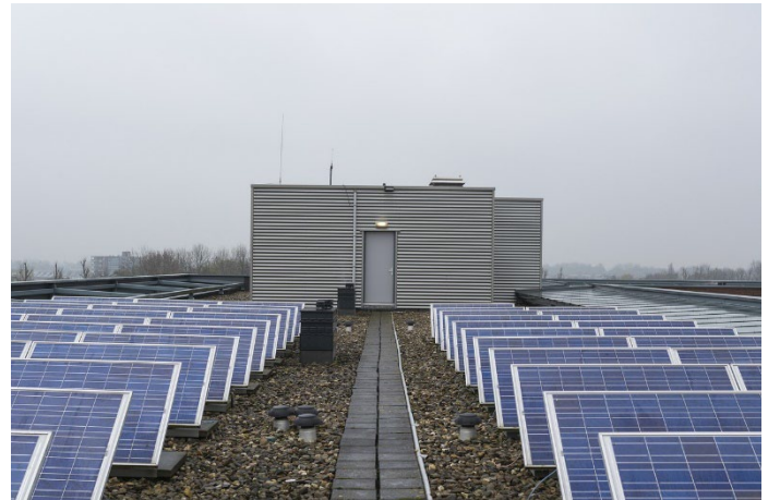
Figure 2: Undamaged lithium-ion batteries may be repurposed in energy storage systems like solar farms.
