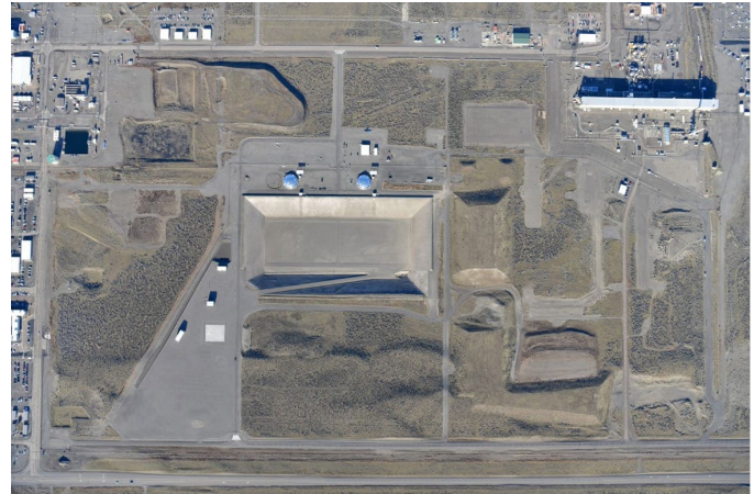
Figure 2. The Integrated Disposal Facility (Photo courtesy of USDOE)
