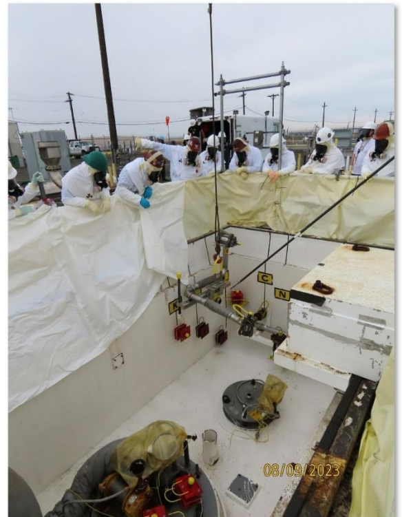
Workers installing waste transfer line
