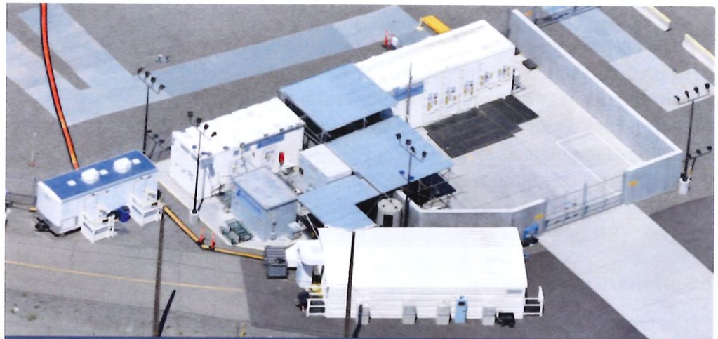
An aerial of Hanford's Tank-Side Cesium Removal System in the 200 East Area.
