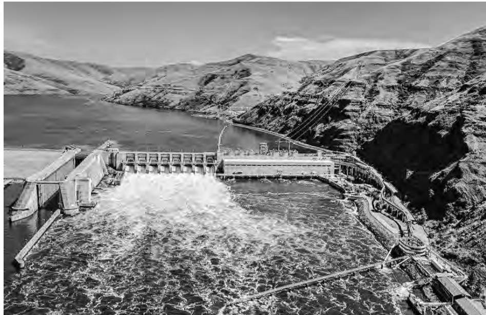
An aerial view of Lower Granite Dam on the Snake River.
