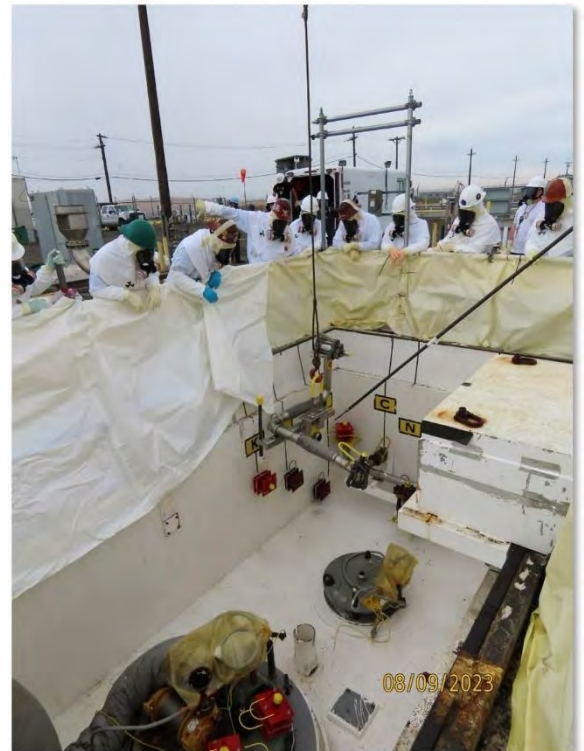
Workers installing waste transfer line
