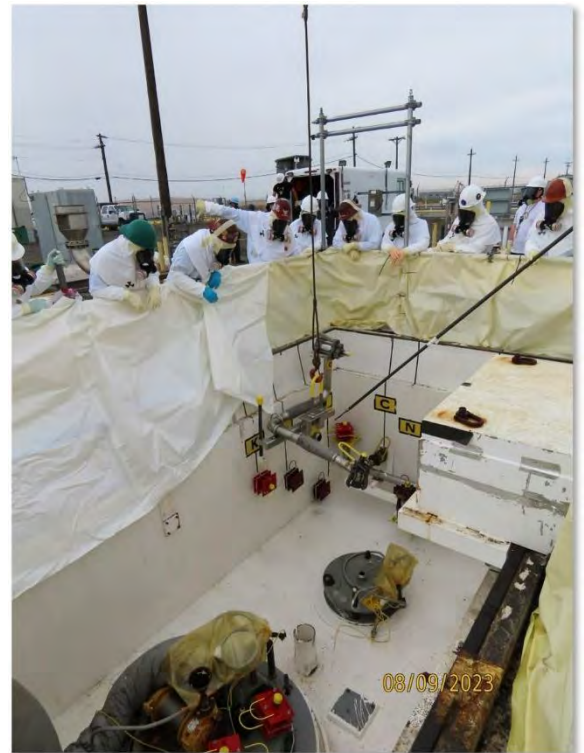
Workers installing waste transfer line
