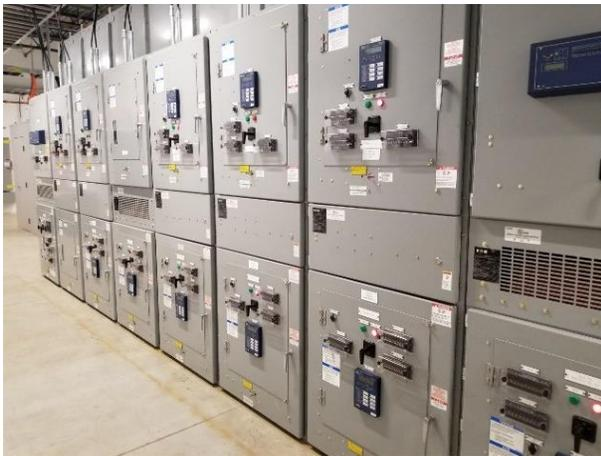
Figure 2-8. Indoor view of switchgear structure
