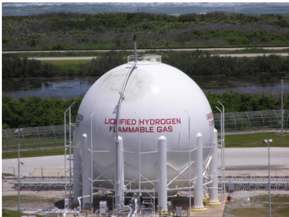
Figure 2-19. Example of a liquid storage tank
