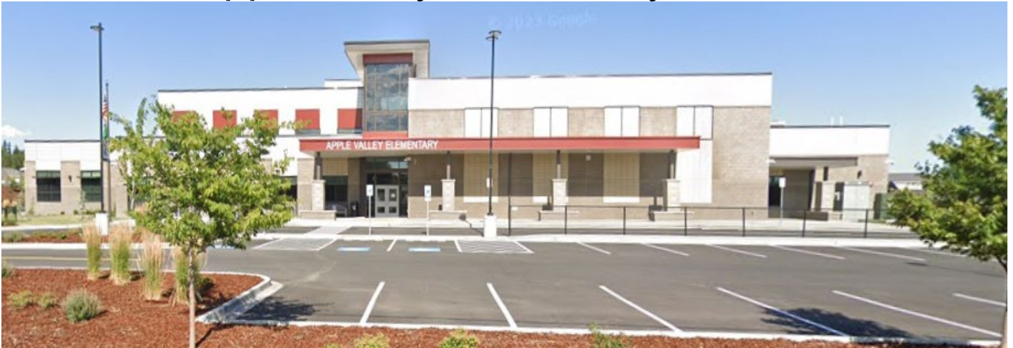
Apple Valley Elementary School – Photo courtesy of Google Street View
