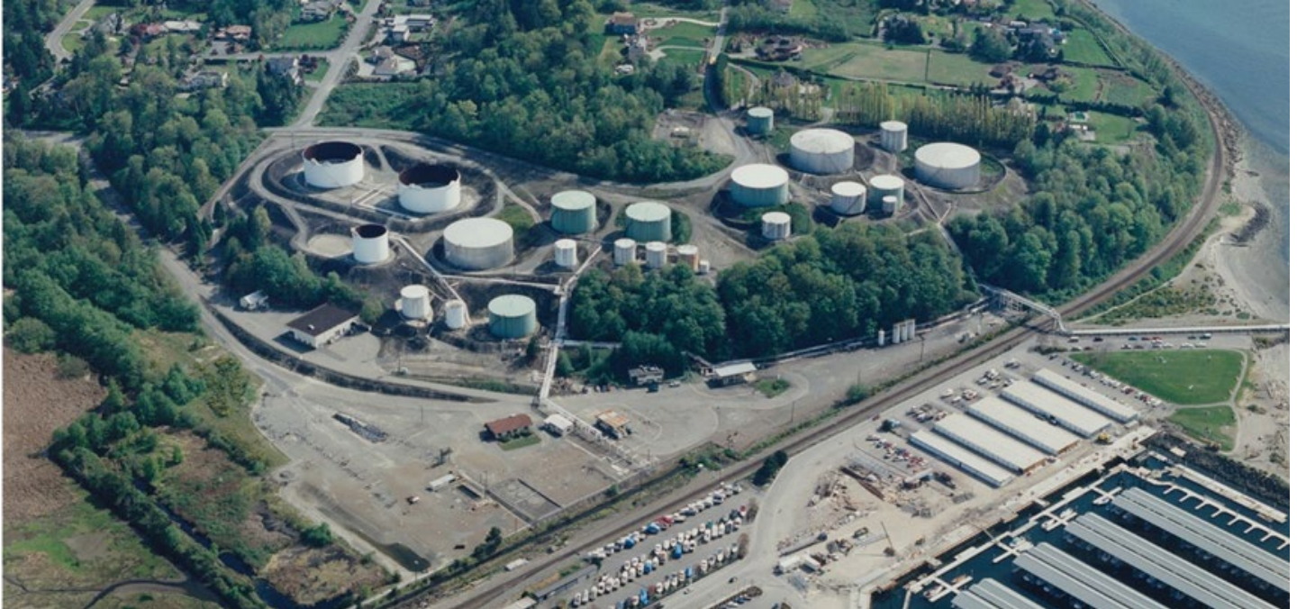
Historic picture of former Unocal Edmonds Bulk Fuel Terminal
