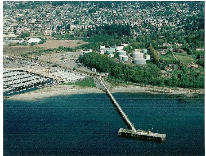
Historic view of fuel terminal
