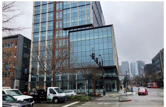
New construction at Block 38 West Property, February 2023
