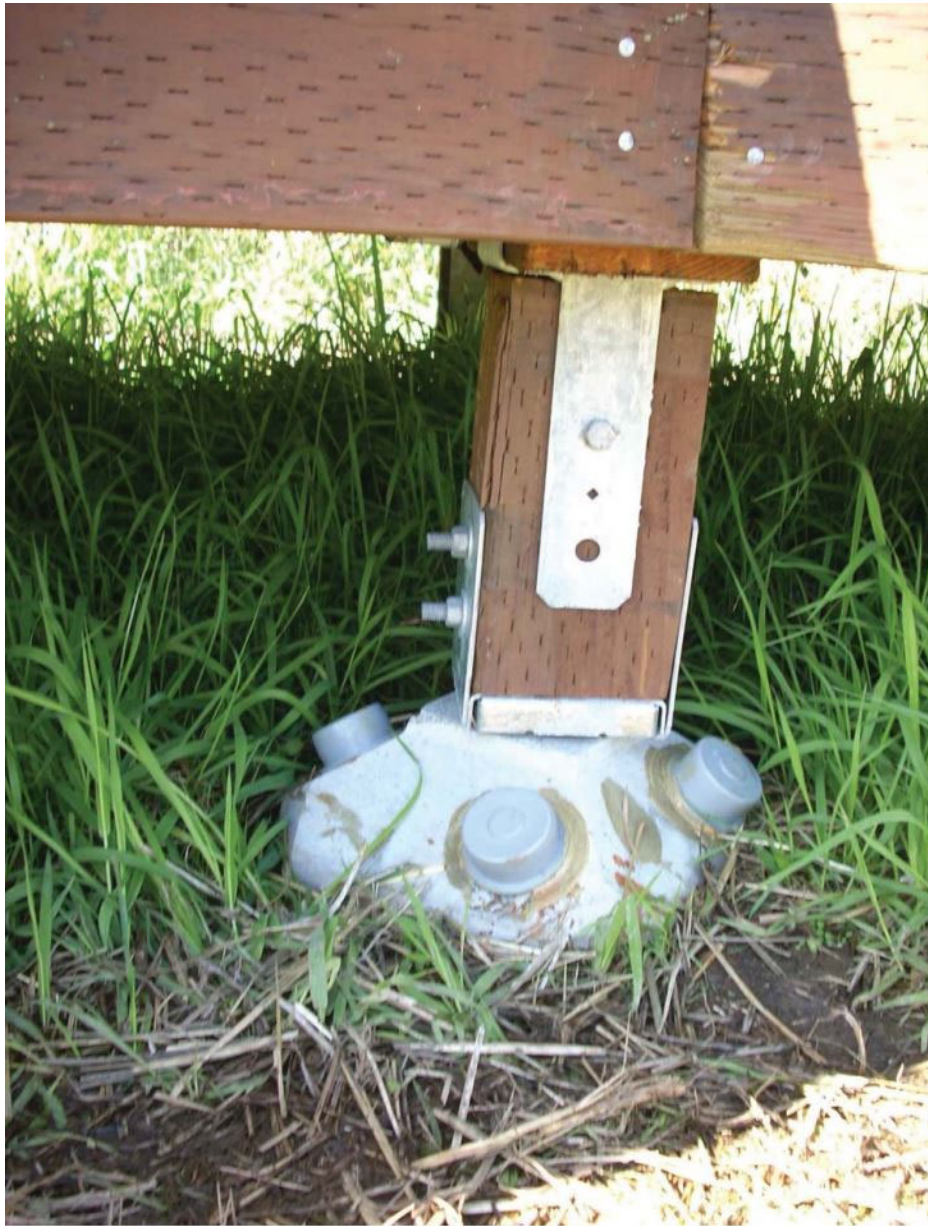
Figure 6.95: Pier-Type Minimal Excavation Foundation
