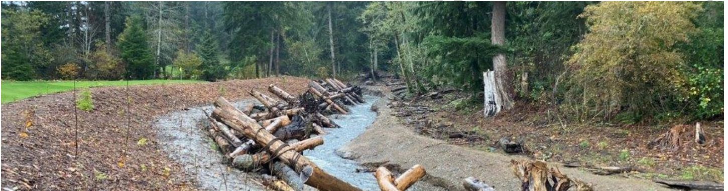
Figure 1. Boise Creek Streamflow Restoration Project
