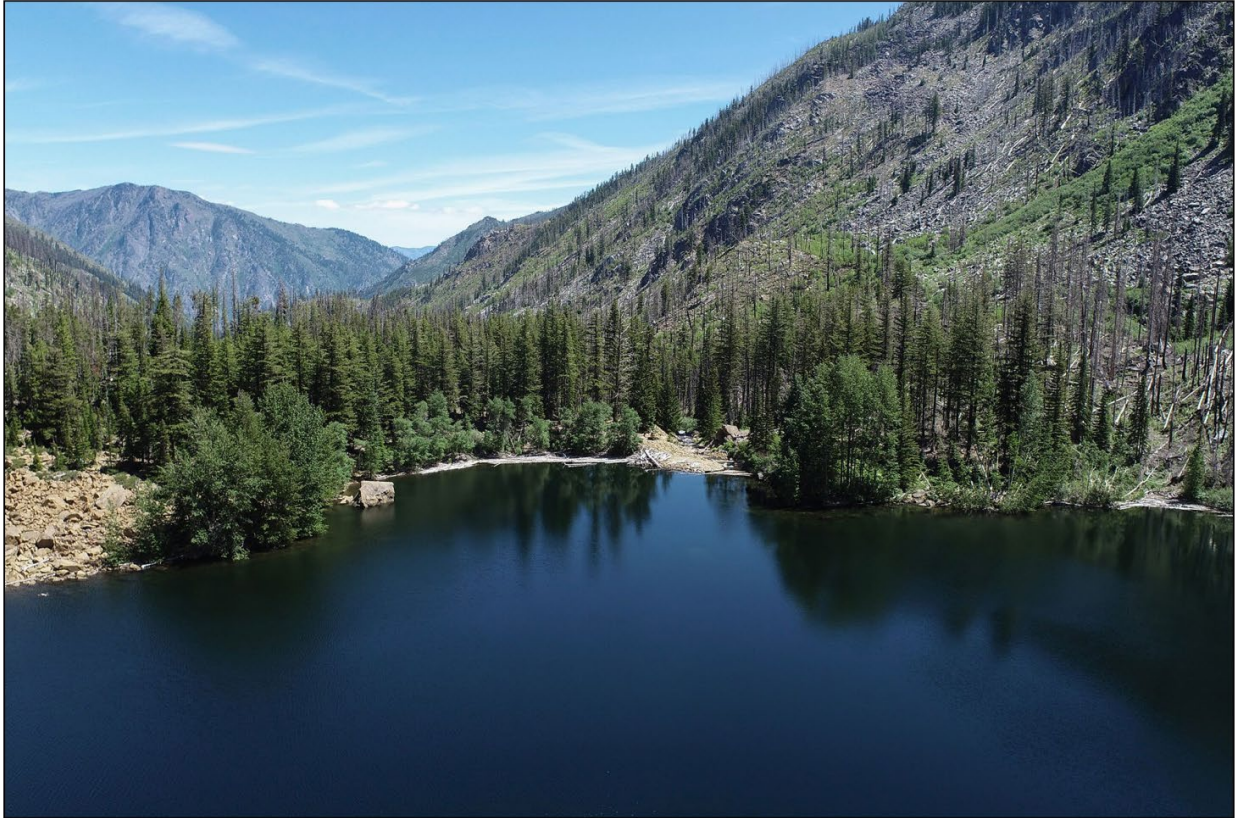
Figure 11-15. KVP C, Aerial Photo of Dam Looking East from Approximately 130 Feet above Eightmile Lake in June 2021
