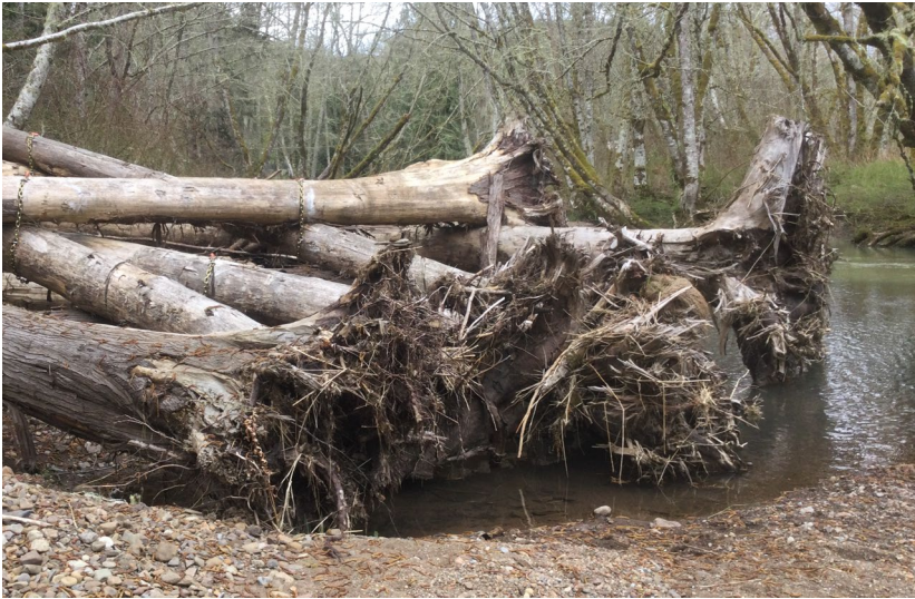
Figure 4. Local scour below root wad logs installed along riverbank
