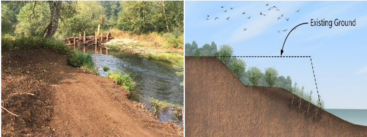
Figure 16. Benching Freshly excavated floodplain bench adjacent to Skookumchuck River. Photograph courtesy Anchor QEA.
