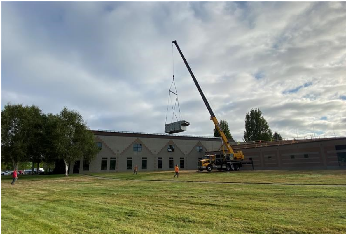
Figure 9: Construction on the Chief Leschi School to improve heating and ventilation. CCA funding enabled this project to give cleaner air to the school's students while also electrifying the old system which reduced emissions. Reducing on-site fossil fuel burning can improve air quality. Photo credit to OSPI.
