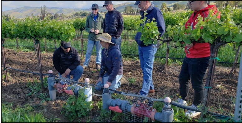
Figure 2. A drip irrigation system on a vineyard in Central Washington. Credit – State Conservation Commission
