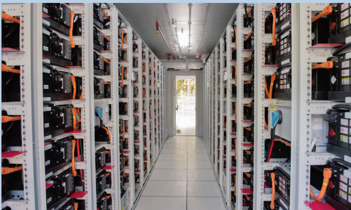
Example of a BESS interior
