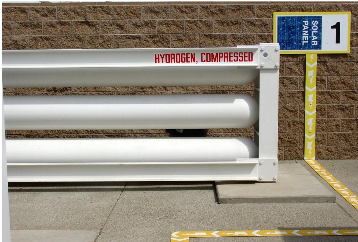
Figure 2-18. Example of a gas storage tank
