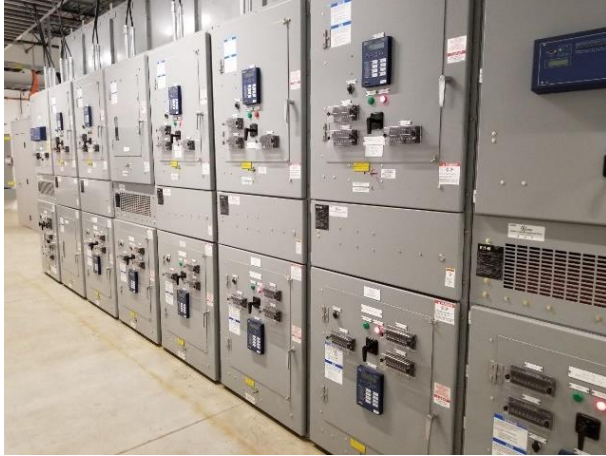
Figure 2-8. Indoor view of switchgear structure
