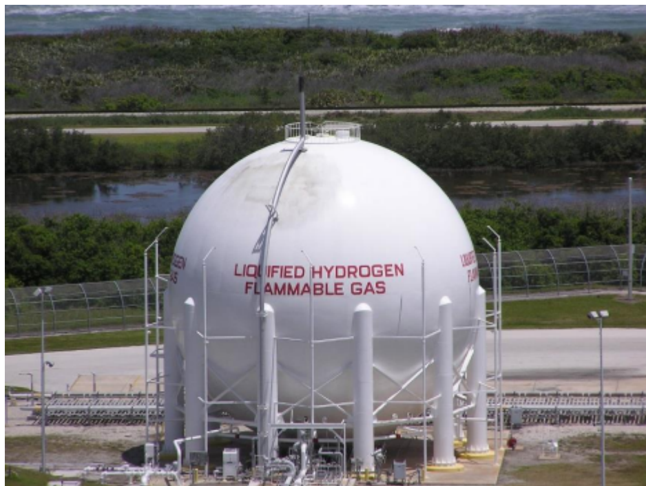
Figure 2-19. Example of a liquid storage tank
