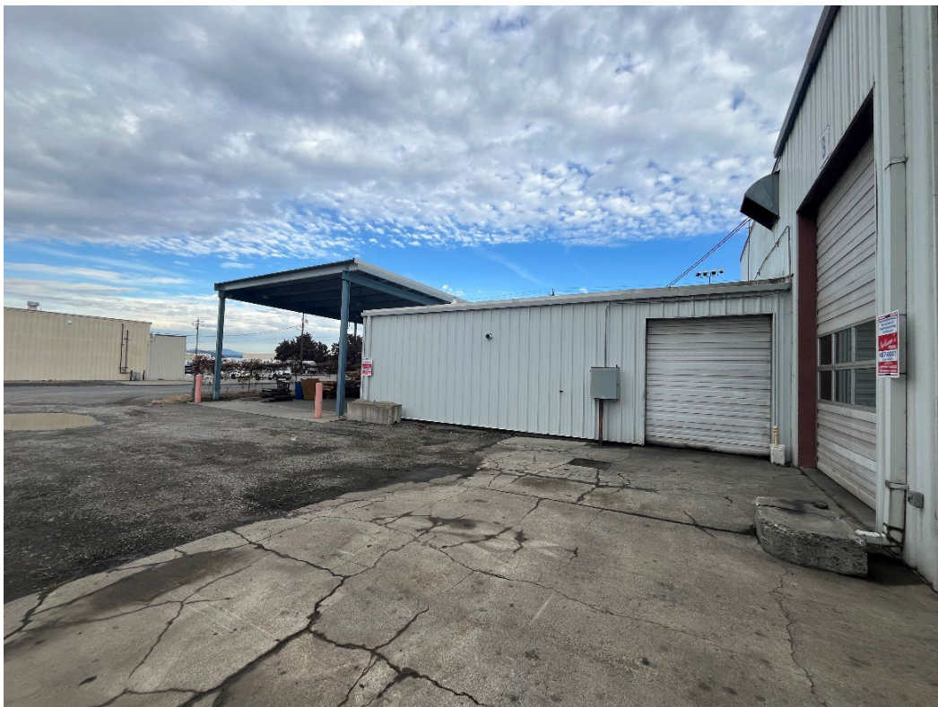
Photo 4: East side of the building — from the west
