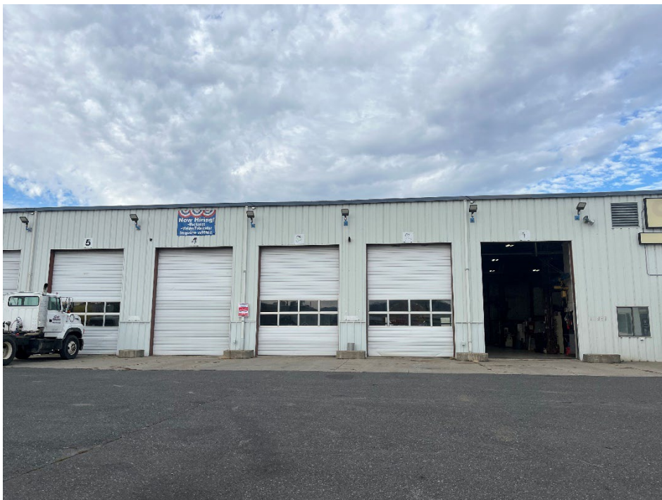
Photo 2: North side of building — from the northeast
