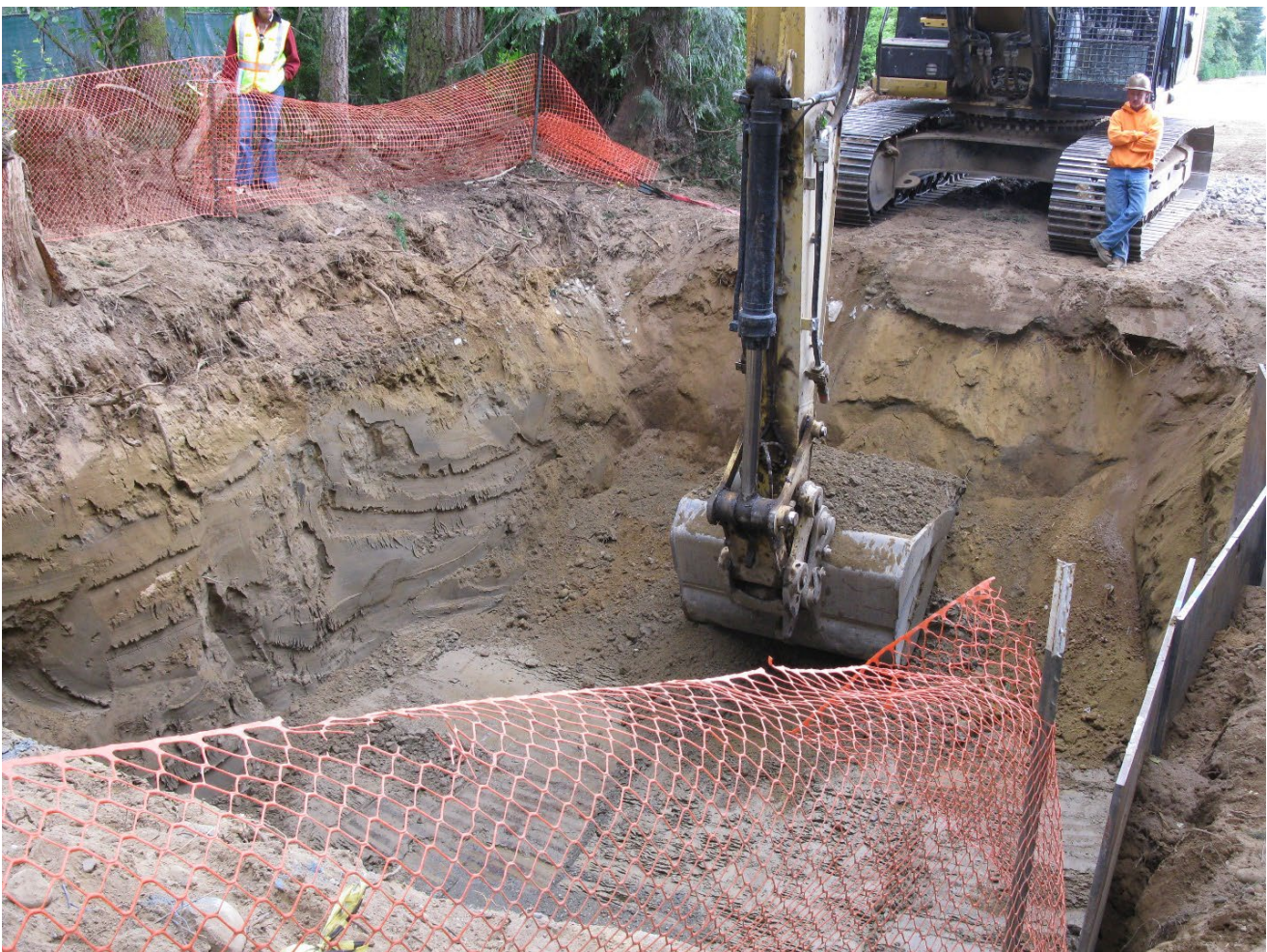
Figure 2. A photo from the excavation work in 2018. Over 10 feet of contaminated soil were excavated from the area behind the warehouse, near the underground storage tank site.
