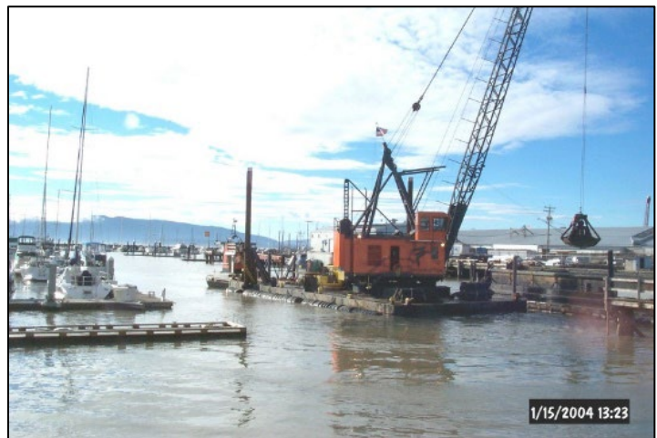
Loading contaminated sediment into a barge during the 2004 interim action
