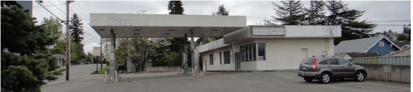
Newman's Chevron Site at 2021 6 th St., Bremerton, WA.
