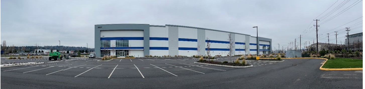
8801 E Marginal Way S cleanup site location
