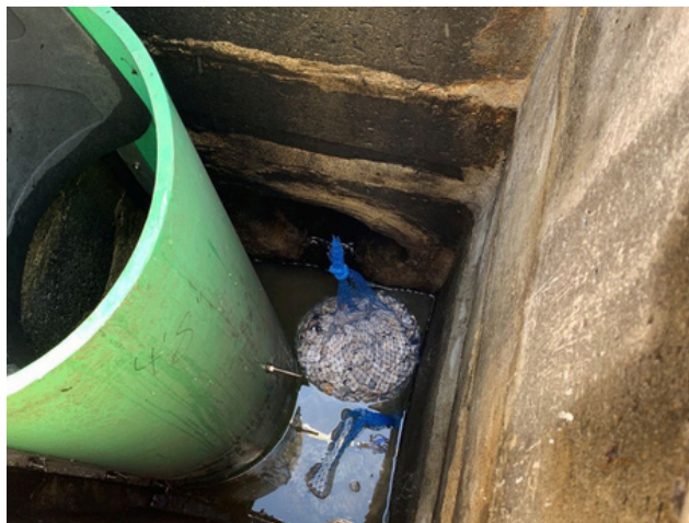
Figure 1. Bagged oyster shells were added to two catch basins.
