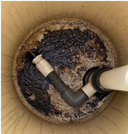
Figure 2: Orifice control on underdrain outlet
