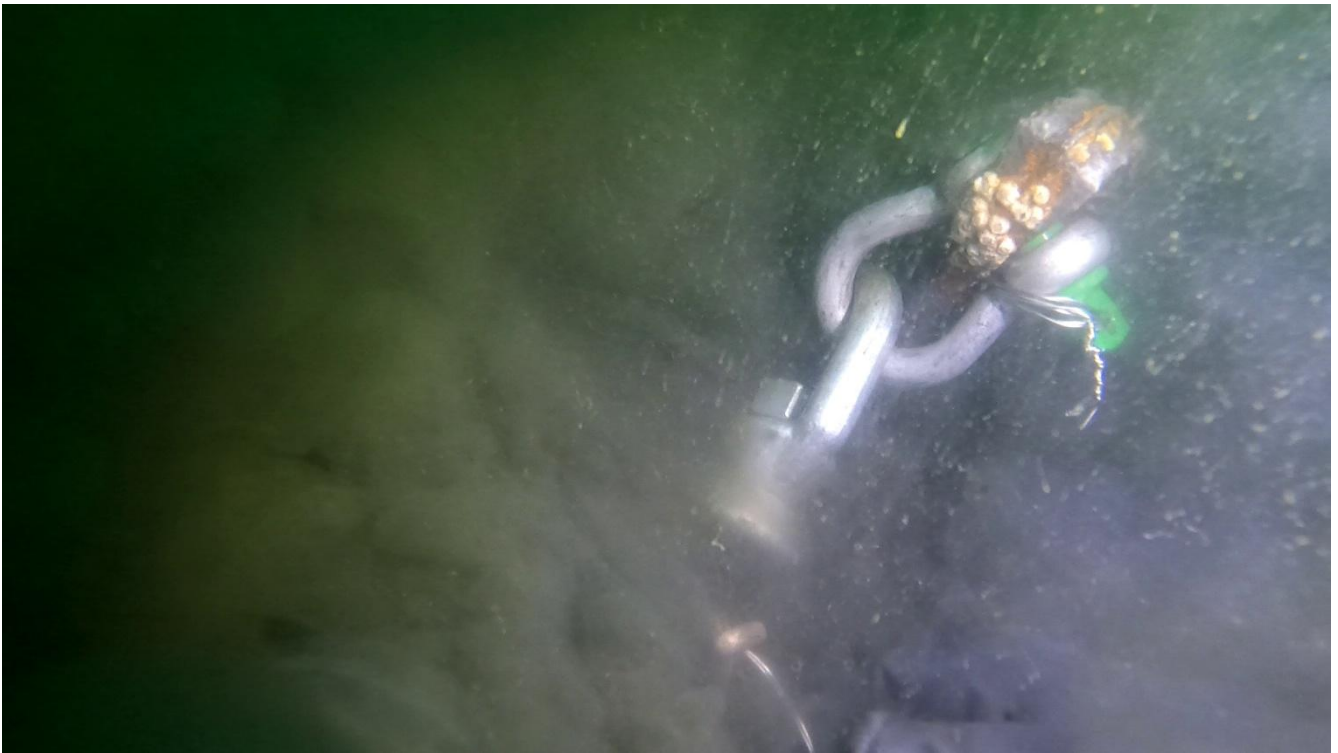
Buoy 3: New anchor shackle & swivel installed.
