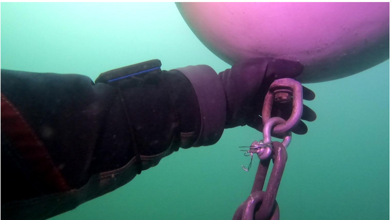
Buoy 1: New midline float, 18" mooring buoy installed.
