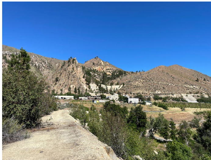
Figure 13: A photo of the tailing impoundment embankment with the Golden King/Lovitt Mine workings in the background.
