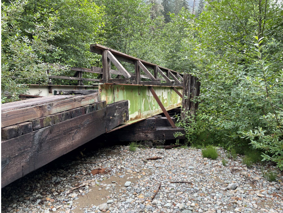
Figure 16: Twin Bridges located in the Monte Cristo Mining Area.
