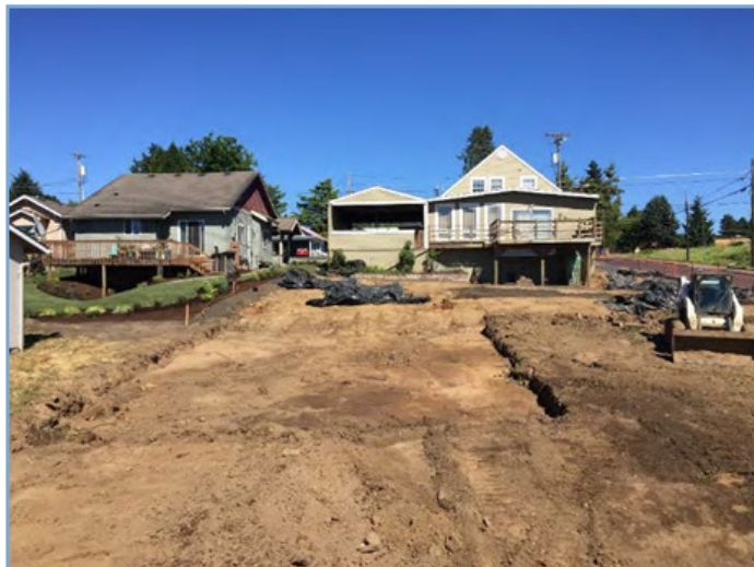
Figure 19: Soil replacement on a property
