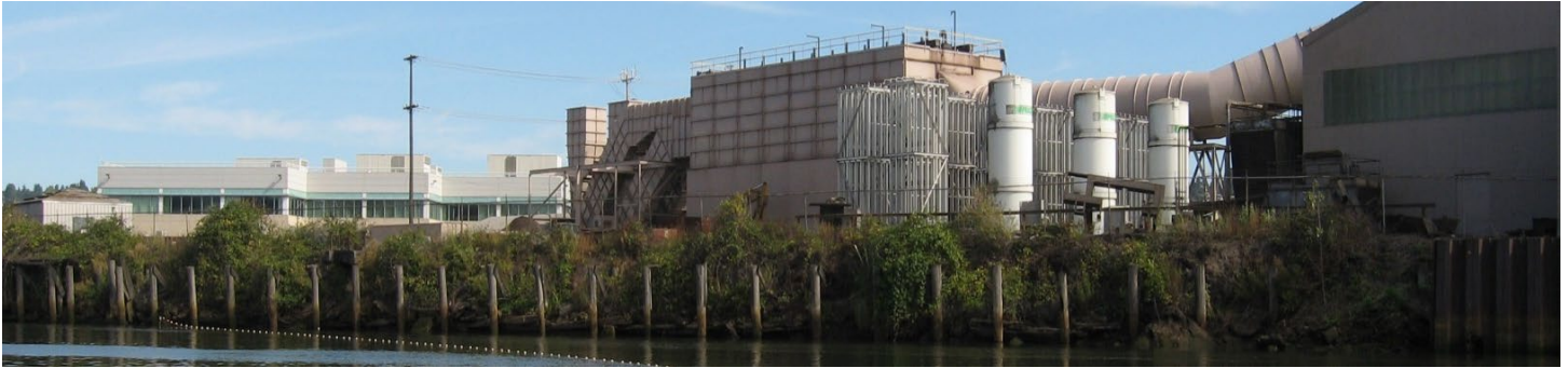
The Jorgensen Forge Corp Site before the buildings were demolished.
